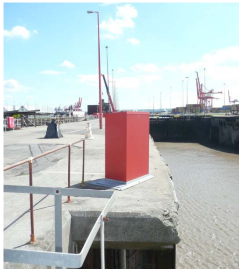
Portbury Tide Gauge Cabinet
