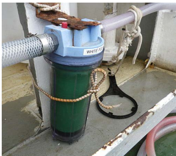
Fig. 17.3 Washing water filter
