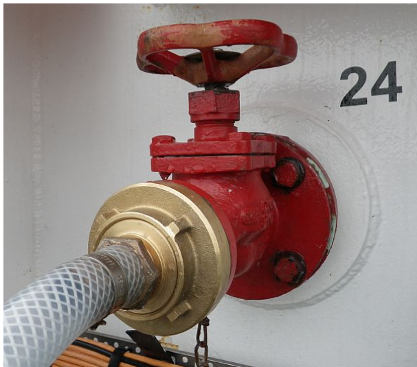
Fig. 17.2 Storz 66 mm firehose coupling with 2.5 cm hose tail connection for seawater.
