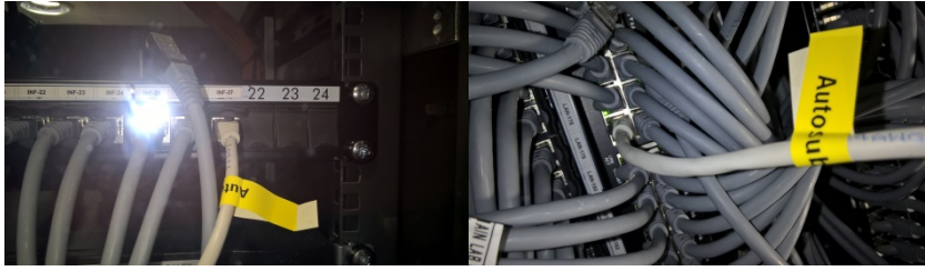
Figure 19.13. INF-R7-25-27 routed to the server room INF-27 Rack 3 bay 1 (left picture) and patched to Main lab socket LAN-179 Rack 3 bay 4 (right picture).
