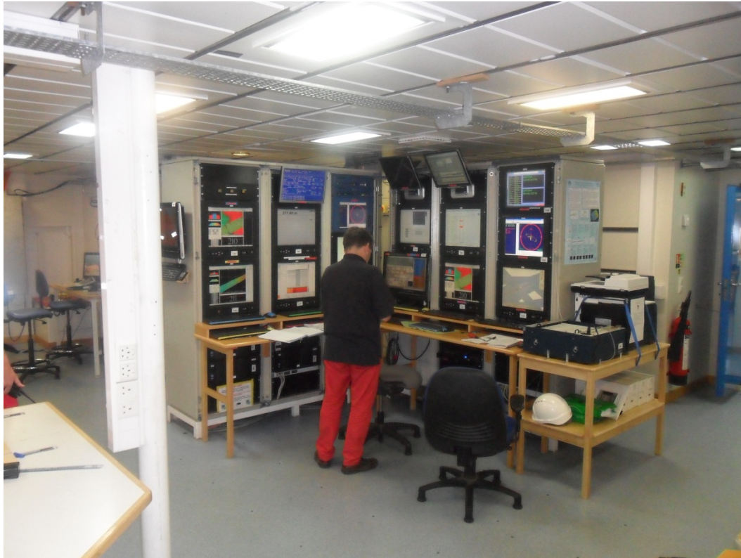
Figure 10. Geophysical and hydrographic corner of the main lab. All scientific equipment including multibeam, sub-bottom profiler, navigation systems, Olex, USBL are rack mounted.
