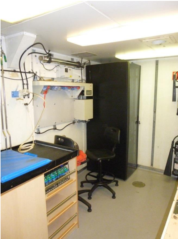
Figure 8.4: rack mounted UWIA in the JCR Prep Lab
