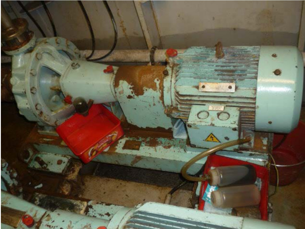
Plate 2: Tangie centrifugal pump used for the UW supply.
