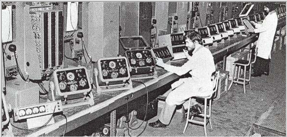
Mk 12 ( left) and Mk 21 (right) equipment is being tested at Decca's Marine Service facility at Croydon, England in the early 1970's. There was a staff of 400 employed at this location. It included workshops, spares inventory, installation, service control, engineering support and training. ( Courtesy Decca Navigator News April, 1972 )
