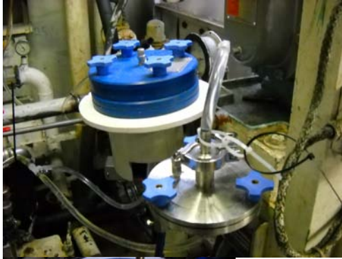
Fig. 2: Underway filtration unit in the engine room
