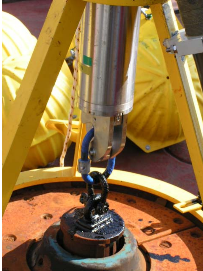
CLOSE VIEW OF RELEASE MECHANISM - SEE ALSO THE ADDITION OF A MODIFIED ANODE TO THE RELEASE LINK - THIS IN DIRECT CONTACT WITH THE LINK NOT INSULATED BY TAPE . MOORING B5
