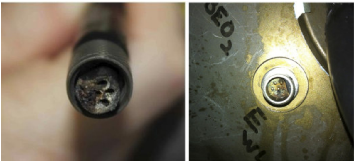
Figure 36: (Left) Photograph of melted plug after blown cable. (Right) Photograph of partially corroded socket.
