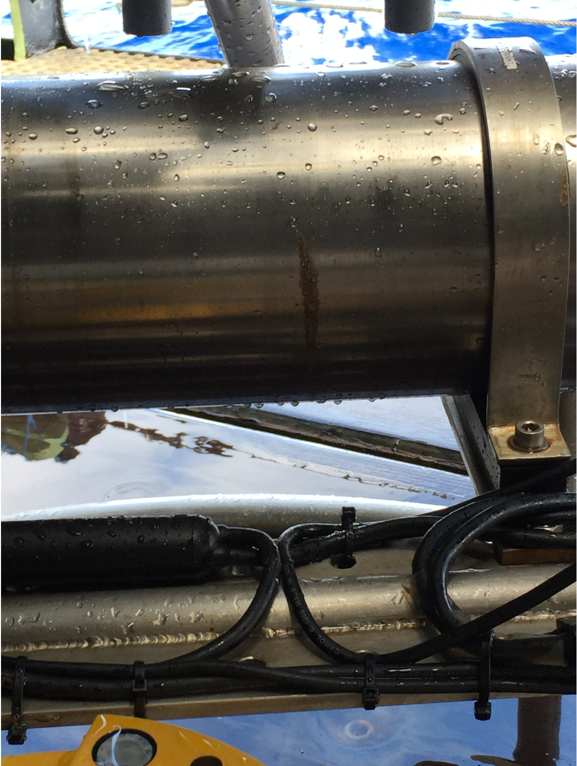
Figure 1.4: LADCP battery pack viewed from inside the CTD frame
