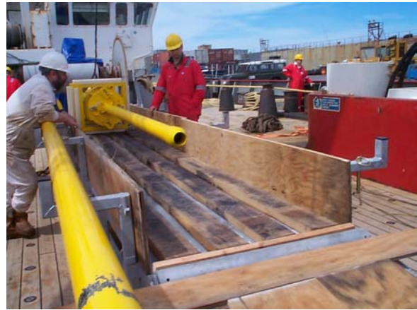
Fig. 11. Plywood sides fitted to the core tables.
