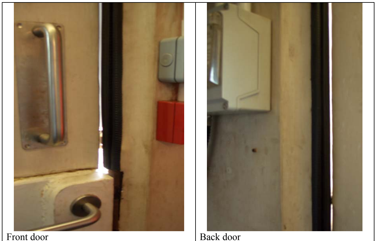
Picture 2, Cracks in door seals
