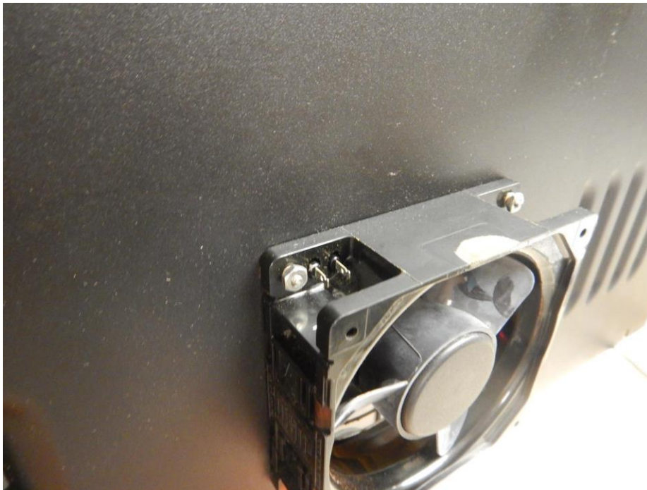
Figure 11:- Autosol S/N 65753 Disconnected Exhaust Fan
