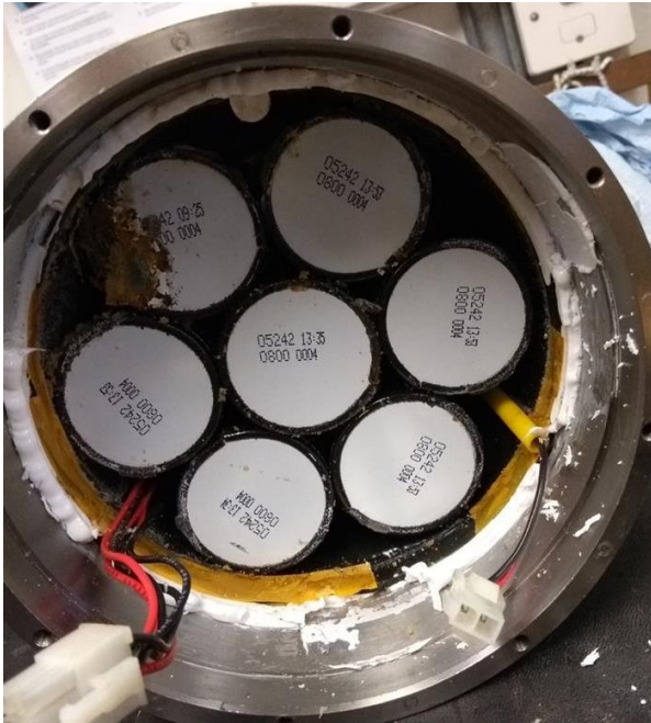
Figure 20:- Chelsea Battery Pack S/N 182042 flooded internals with corroded batteries
