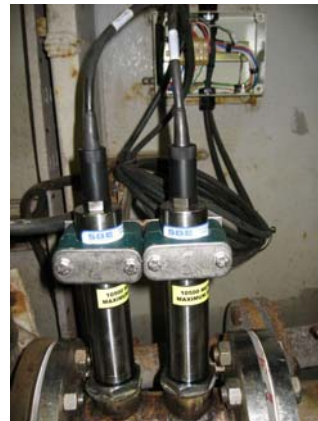
Figure 9. The support bracket needs to be rectified. It is out of alignment when the sensors are fitted and you cannot tighten it properly without adding stress to the installation. The support wants cutting off, and re-welding with everything bolted up leaving a slight gap between the flat-bar and strut it bolts too, to allow fitting of a rubber-shim to give some dampening/tolerance.
