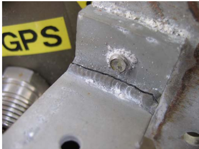
Figure 39. Failed weld on upper starboard tail frame section
