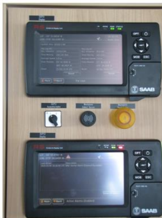
Figure 12. GPS1 and GPS2 displays on bridge.
