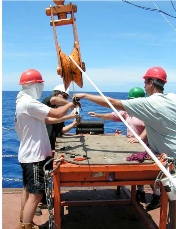
Photograph C.6: Mooring Table – Attaching an SBE37 Microcat
