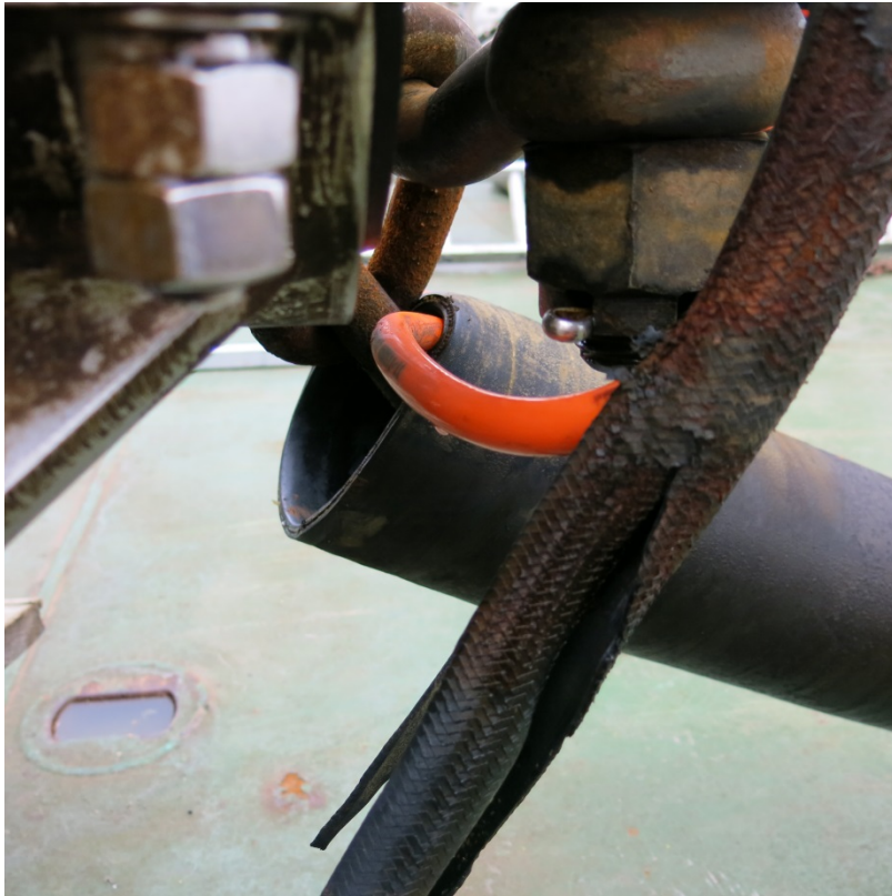
Figure 24: Orange cable near the frame-chain connection
