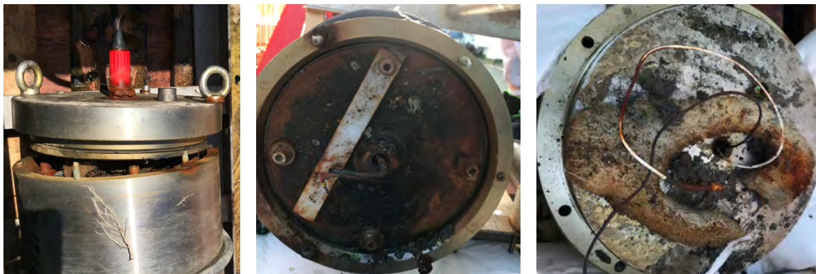
Figure 12.4 Battery housing SN07 on recovery. Bolts have sheared off to open the lid, likely caused by seawater leaking into the housing and reacting with the lithium batteries.
