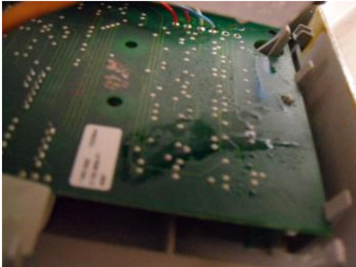
Figure 6.15: Photograph showing the condensation on the internal circuit board of one of the thermocirculators immediately after being removed from its internal casing in the Cool Spec room (condensation is shown by where a finger has been drawn across the board)
