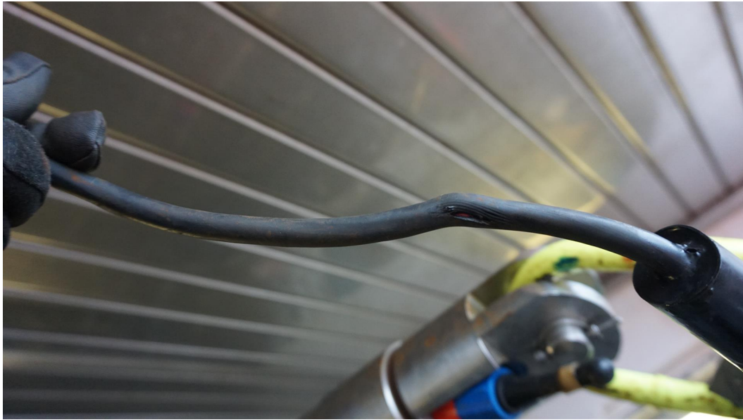
Figure 48: Damage to tail on conducting wire
