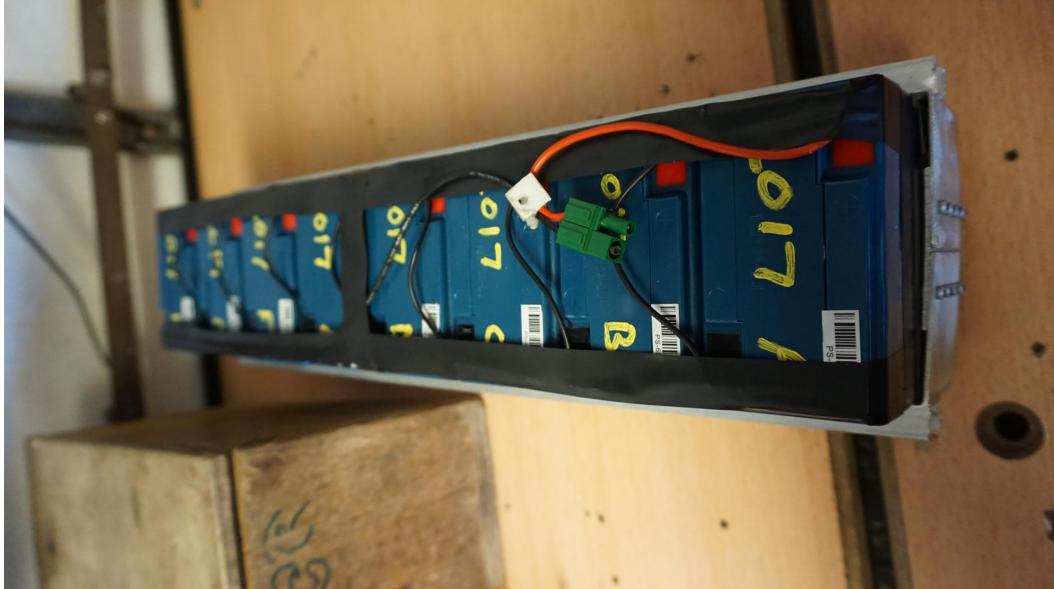
Figure 54: LADCP battery housing wiring prior to modification
