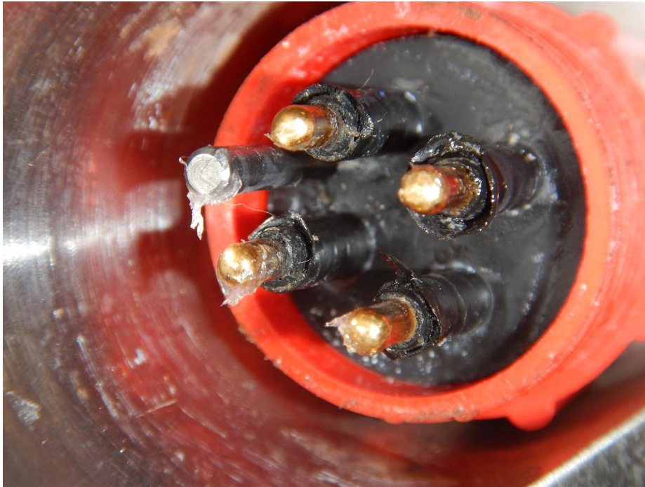
Figure 50: CTD Swivel damage to rubber seal on pins
