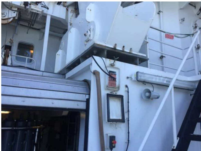
Figure 2.3c SUCS power setup in CTD annex
