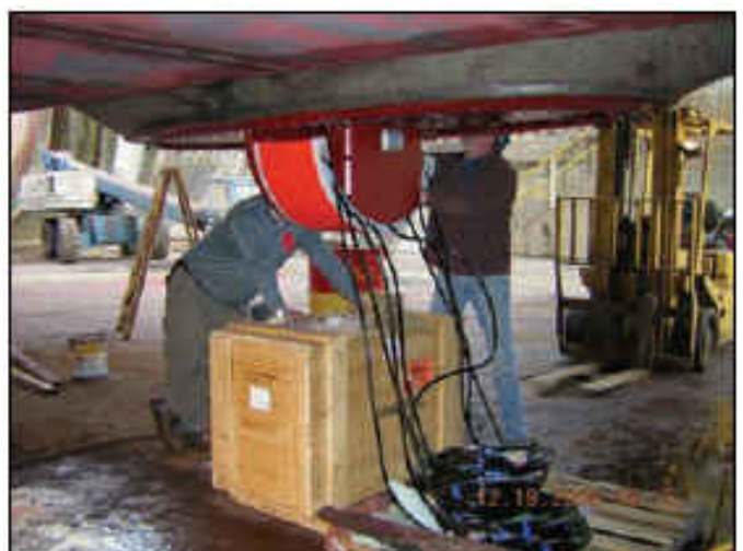
Fig 2: EM1002 transducer
