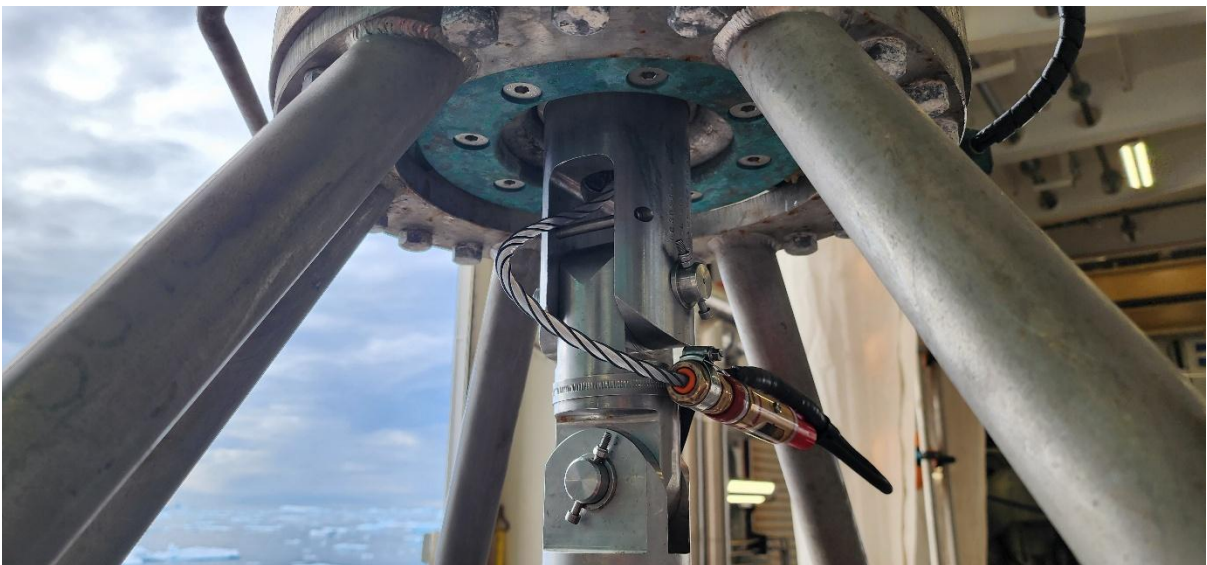
Figure 7.2-16. New OFJB after re-termination.
