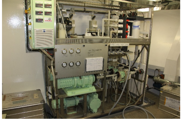
Evaluated flow-through system (Underway system) on board RV SONNE.
